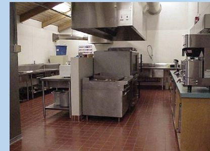
TFCC commercial kitchen
